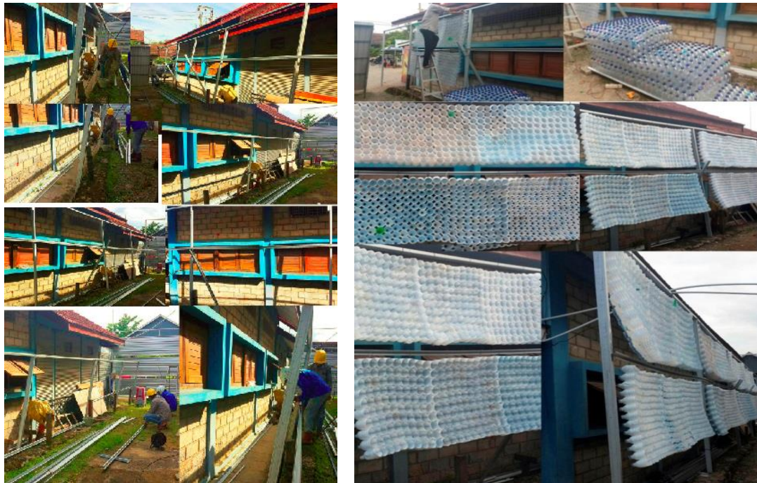
Figure 3B. Implementation of plastic bottle waste as a building envelope
