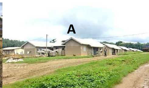
Photo 7: Newly Constructed Workers' camp 'A' at Penda Mboko
